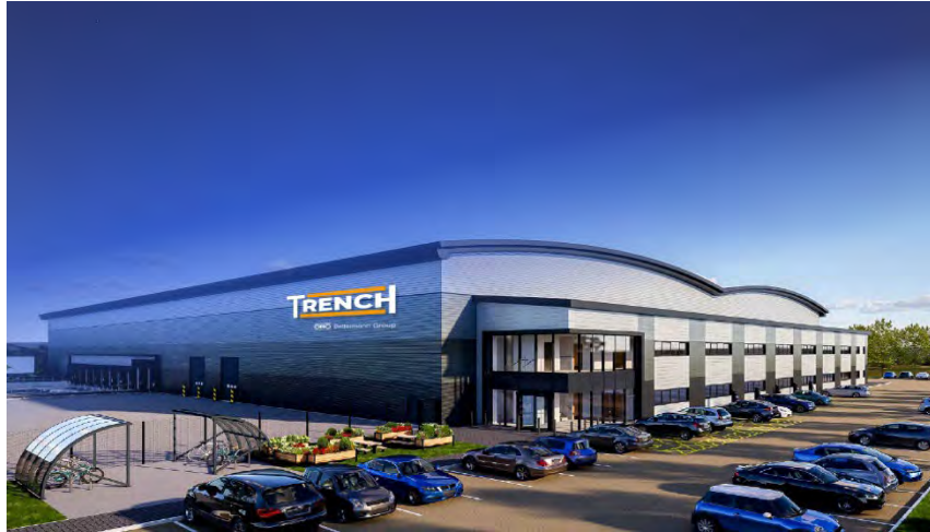
Trench Ltd (UK) 10,000 m 2
