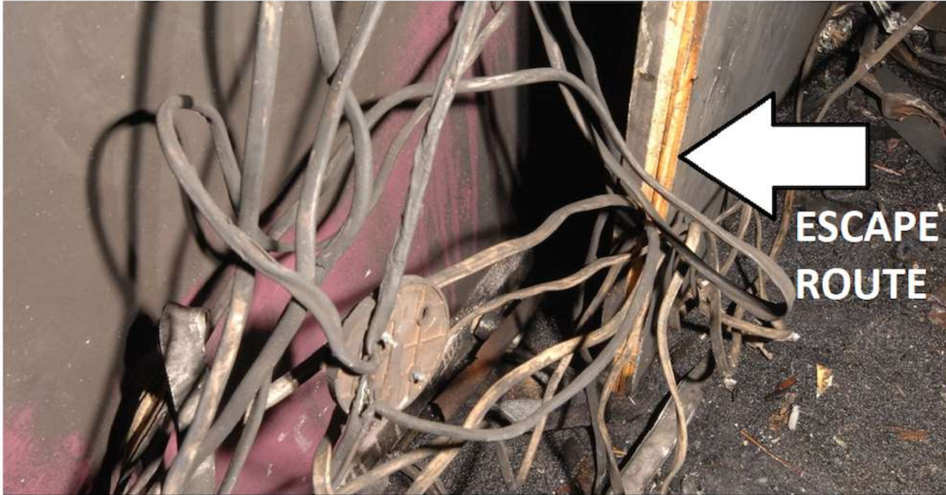
Jim Shears and Alan Bannon lost their lives in the blaze at Shirley Towers. The inquest into their deaths has heard they became tangled in fallen cables.
